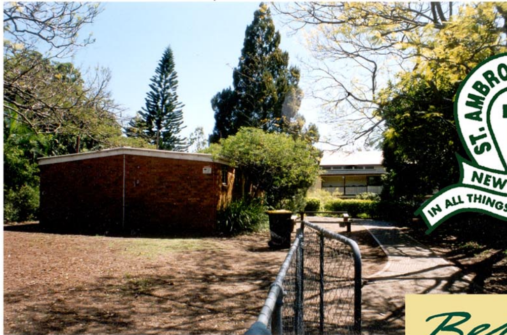
NORTH VIEW OF STAGE 3 (FROM STAGE 1 BUILDING)
